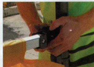
3. Insert half wall bar into connector and tighten the connector. Repeat for both sides.
