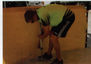
6. Adjust the height of the support leg until securely in position.
