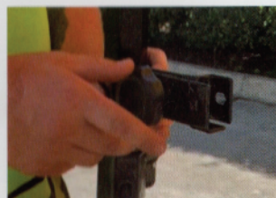
1. Attach half wall connectors to frame legs above the push button leg connectors.
