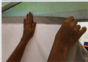
1. Attach walls to roof along Velcro strips.
