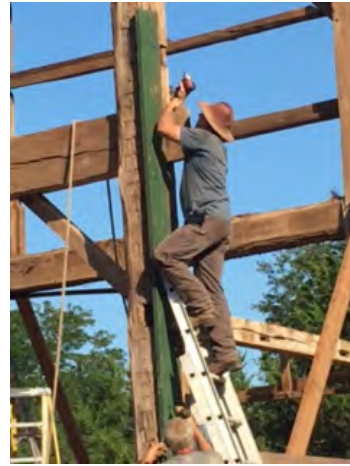
Restoration Technologies Principal Adam Wengryn steadying a fragile beam before the barn bent is lowered
