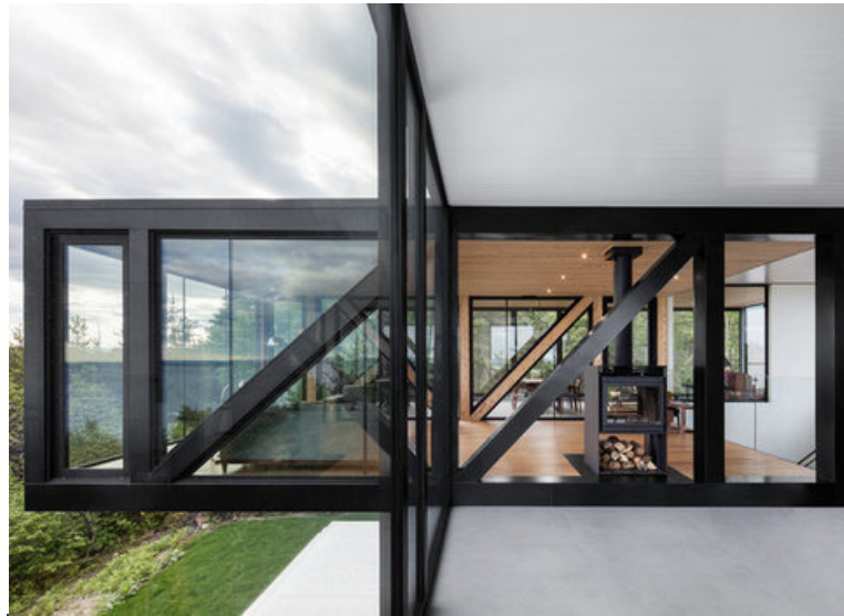
ARCHITECTURAL , INTERIOR AND EXPOSED STEEL FRAMES
