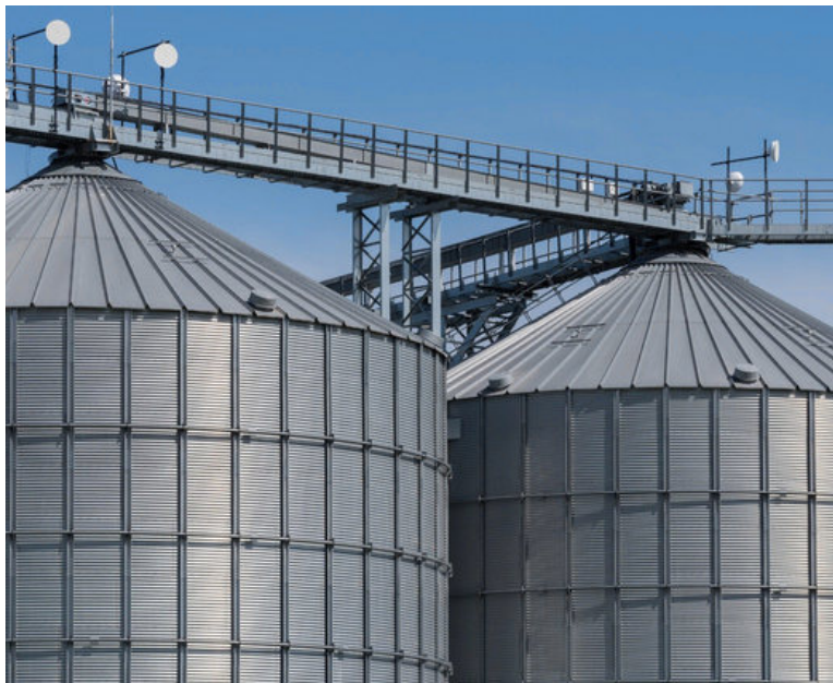
CILOS AND STORAGE TANKS
