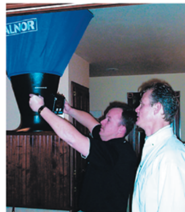
Thompson Homes, Inc., makes sure moisture is removed from bathrooms using a ventilating system that is tested and certified by the Wisconsin ENERGY STAR Homes Program.
