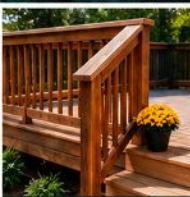
DECKS & OUTDOOR Repairs & Upgrades.
