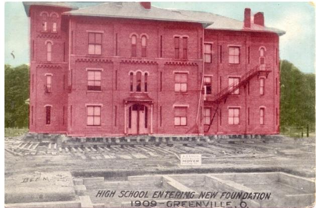
Moving the old West High School from its old location in the center of the block to the west side of the block along Central Avenue in 1909 to make way for the new Memorial Hall (above-colored post cards from 1909 showing the building raised onto logs, then moved to the west).
