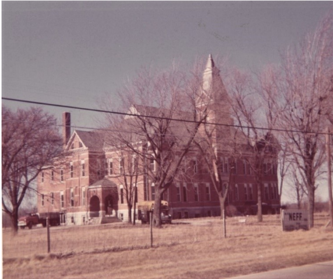
March, 1972 getting ready for demolition
