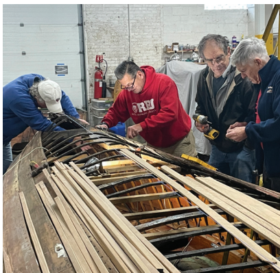
Installing New Ribs
