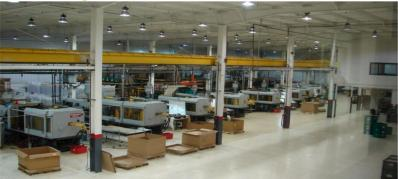
91 High bays,400w MH - 120 watt LED 8 Wall pack, 400w MH - 80w LED 9 High bays,400w MH - 18.5 watt LED
