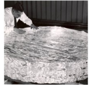
Corning flame hydrolysis fused silica boule process circa 1960's.
