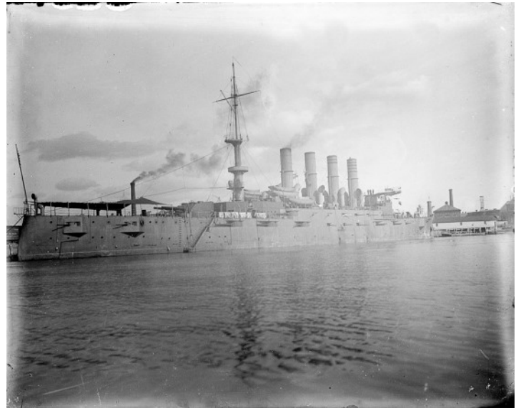
First Class Cruiser either Pennsylvania Class or Tennessee Class. Length 504 ft Beam 69.5 Ft
