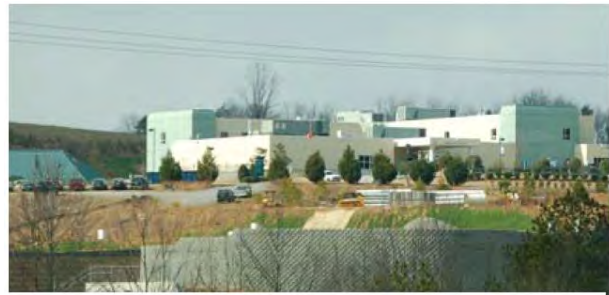
Piedmont Mountainside Hospital
