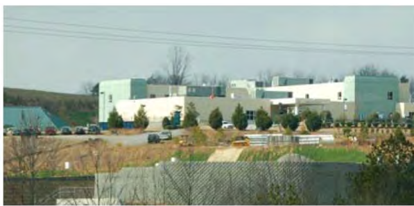
Piedmont Mountainside Hospital
