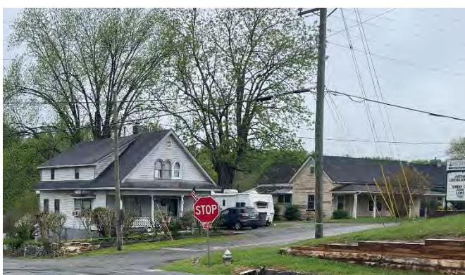
Figure 71: Historic single family detached residence.
