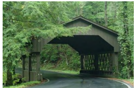
Figure 38: Covered Bridge inside Big Canoe
