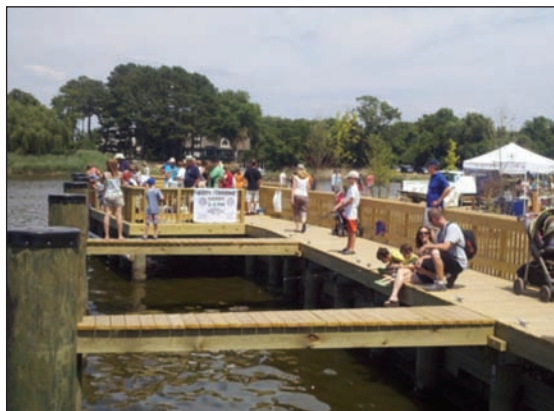
New Centreville Wharf fishing pier, finger piers, and boardwalk
