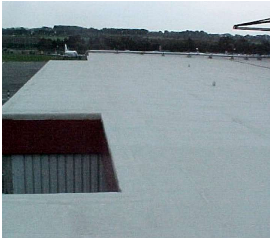
Airport fire station roof repair
