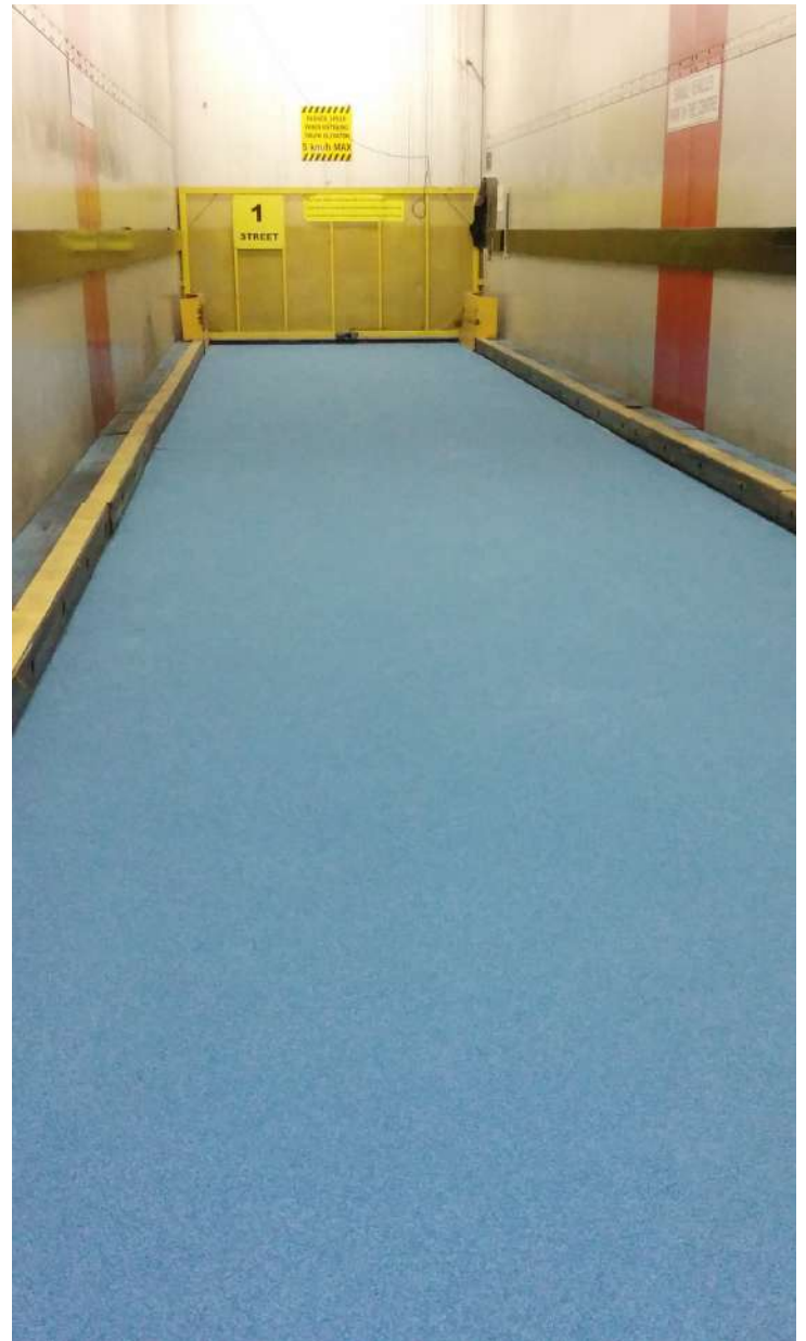
Commercial truck lift floor repair and protection
