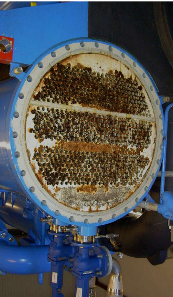
Tubesheet repair at an airport
