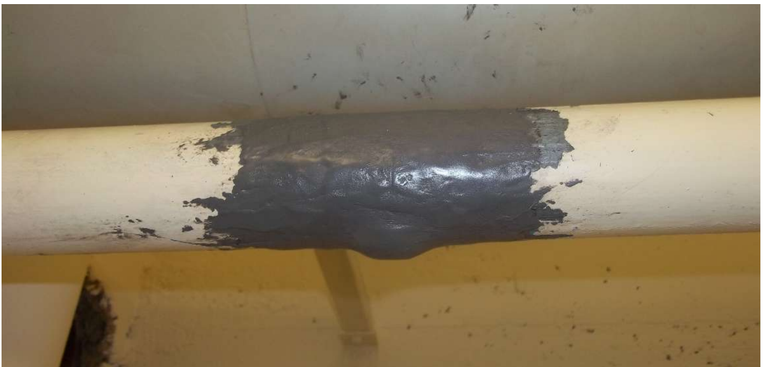
Emergency pipe repair
