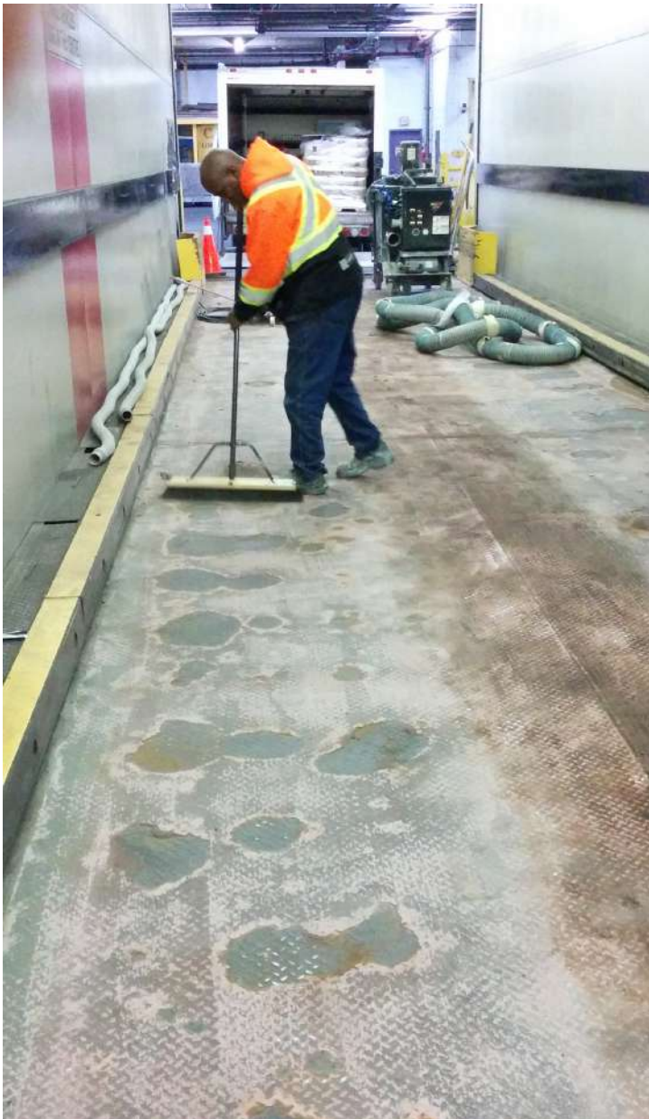
Commercial truck lift floor repair and protection
