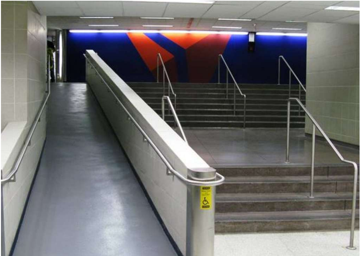
Wheelchair access ramp floor repair at an airport
