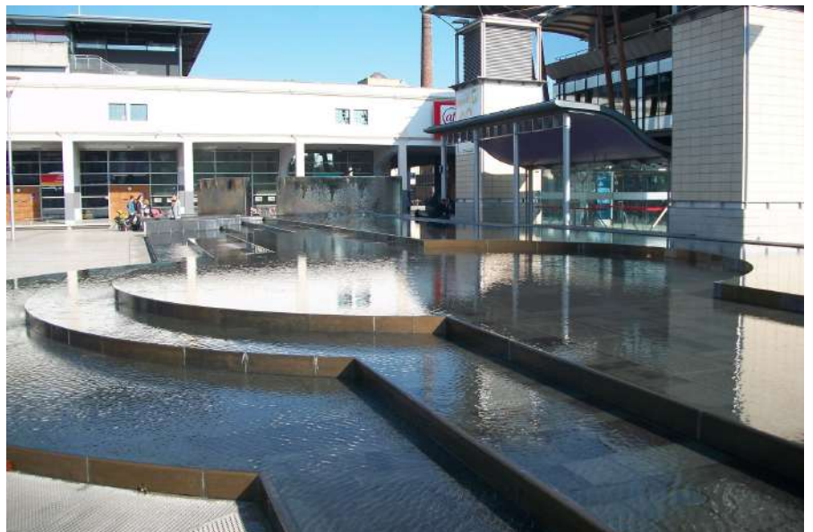
Completed fountain application
