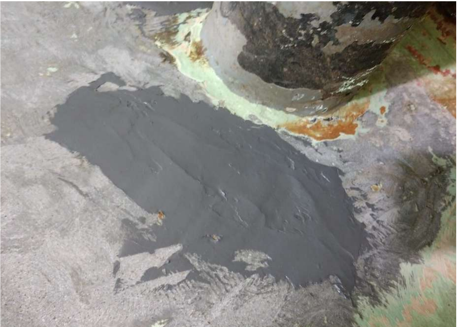
Leak sealed on a wastewater holding tank
