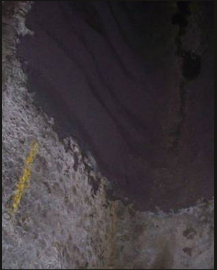
Trough fully coated with Belzona 1812
