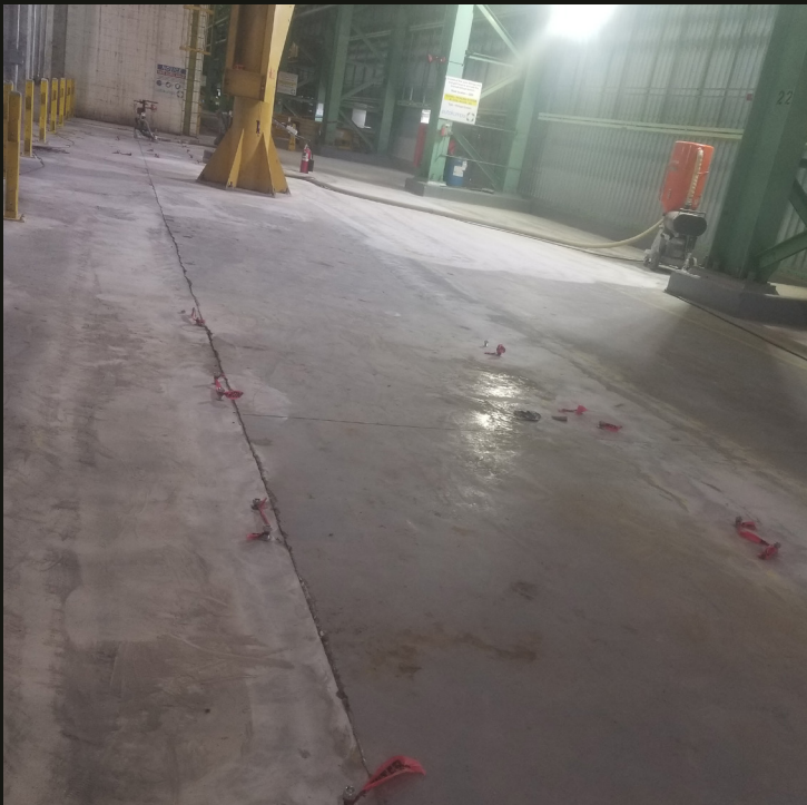
Before: A facility floor without slip-resistance
