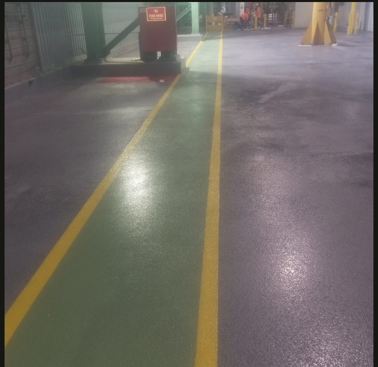
After: Belzona slip-resistant floor system (Belzona 5811 with Belzona 9211 aggregate) installed.
