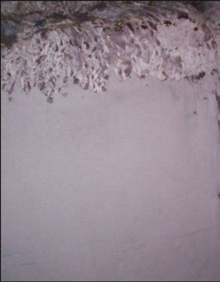
A further quarter inch of Belzona 4111 applied
