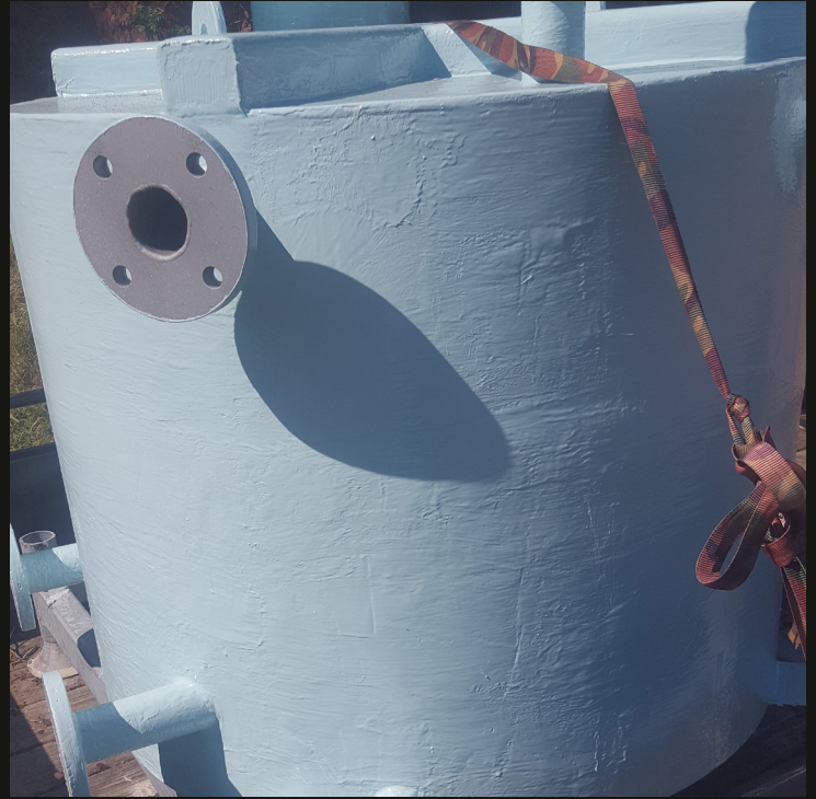
After: A condensate tank reprofiled with Belzona 1111 and coated with Belzona 1593
