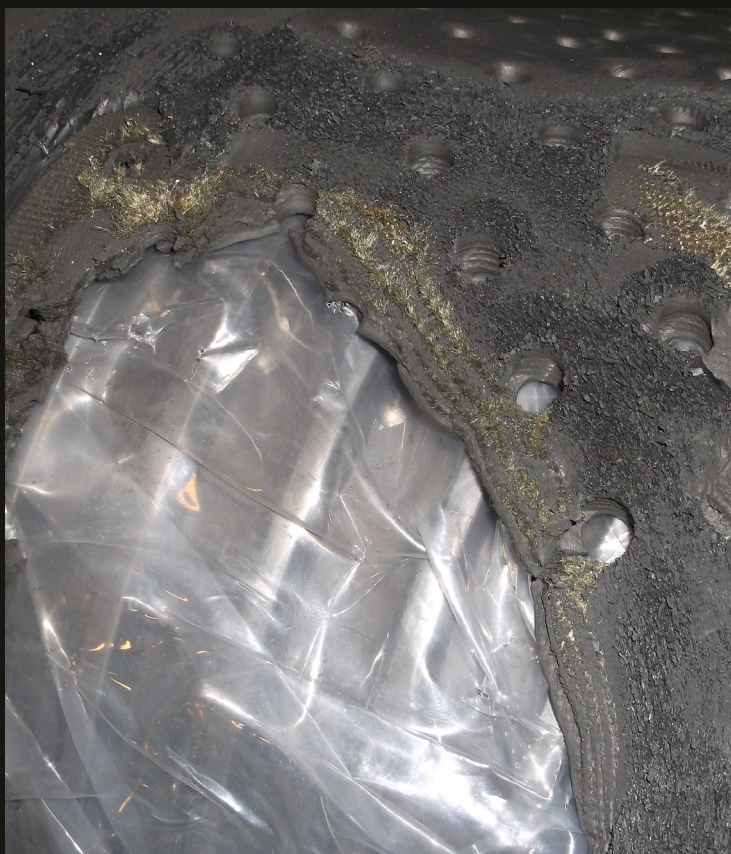
Roughened up area ready for application
