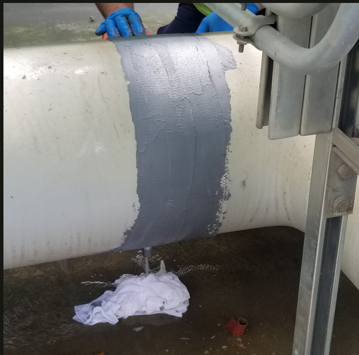
After: Live pipe leak repaired using Belzona 9611, Belzona 1212, & Belzona 9411 reinforcement sheet
