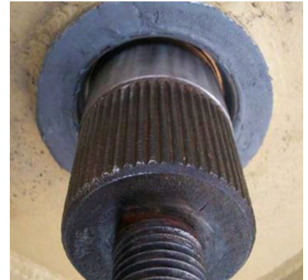
Bearing bushing rebuilt in situ
