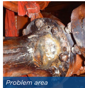
Live leak sealing
