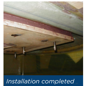
Close up of bonded area
