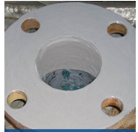
Rebuilding application completed
