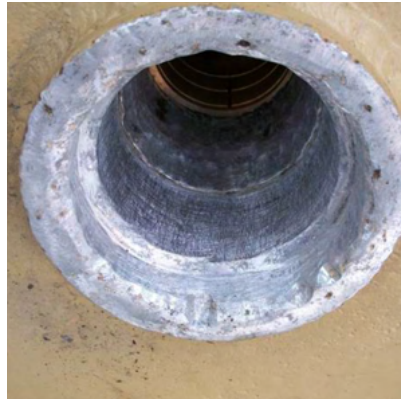
Damaged bearing bushing
