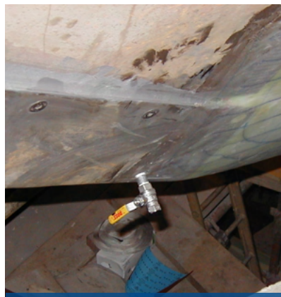
Anchor pocket bonding in progress
