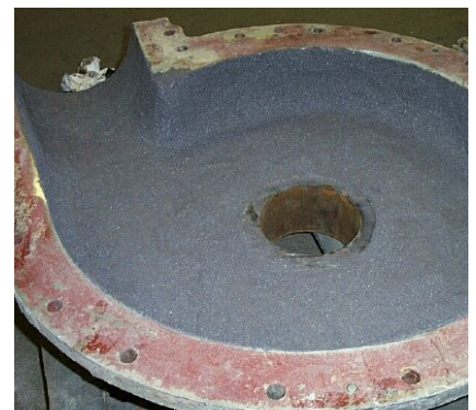
Abrasion resistant coating applied
