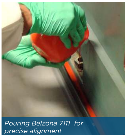
Newly installed equipment requiring chocking
