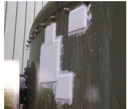
Tank repaired by cold bonding
