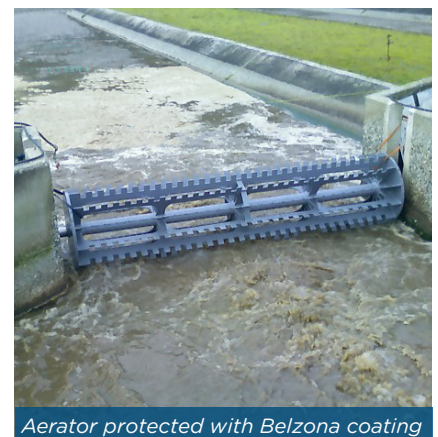
Rebuilt and protected against abrasion
