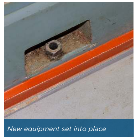
Belzona 100% solids chocking compound applied
