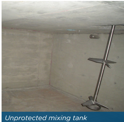
Tank showing severe corrosion
