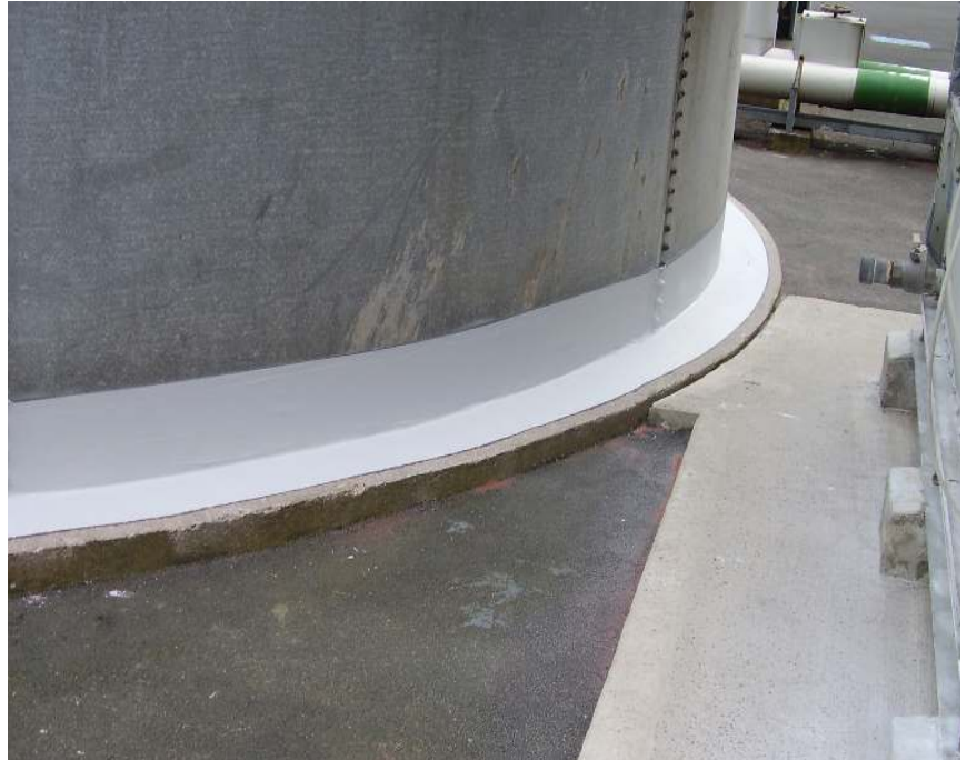
Belzona lining applied to a newly fabricated process vessel
