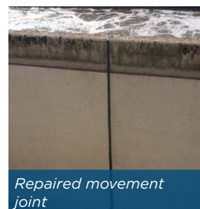
Expansion joint sealed with Belzona material
