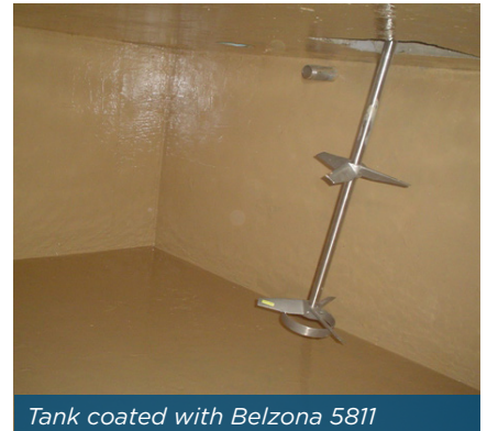
Tank lined with Belzona 5811
