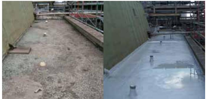
Sealed flashing at roof/wall interface
