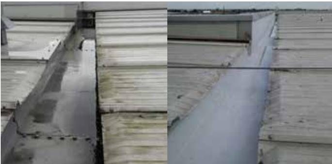
Damaged gutter seamlessly sealed
