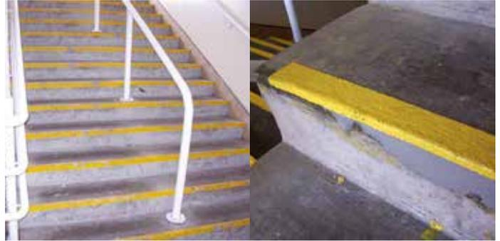
Worn step nosings rebuilt
