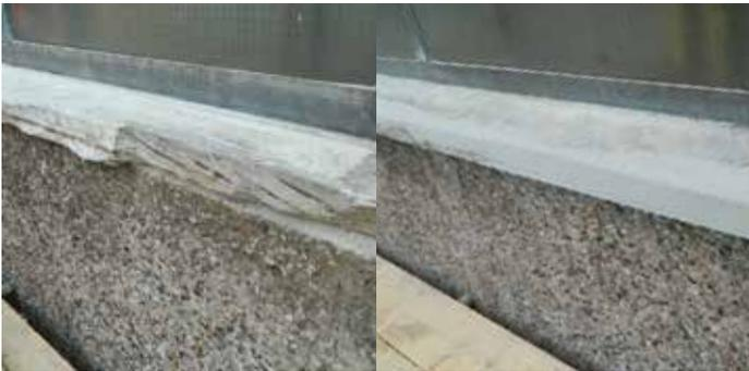
Spalled concrete window sill repaired
