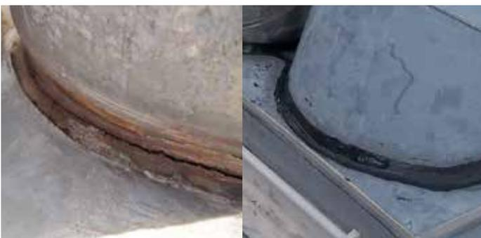
Deteriorated HVAC joints sealed
