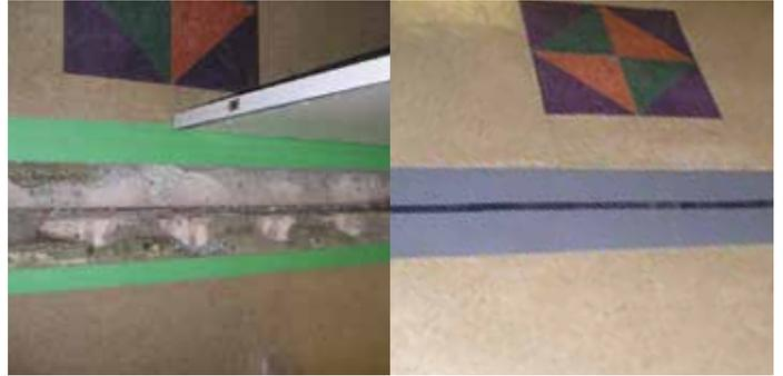
Failed expansion joint in hospital repaired
