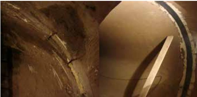
Joints sealed on underground concrete pipes
