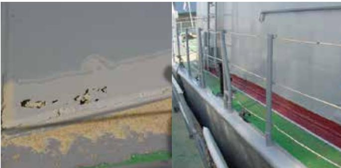
Joint between deck and vessel sealed
