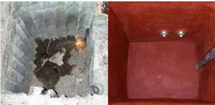
Sump rebuilt with chemically resistant material
