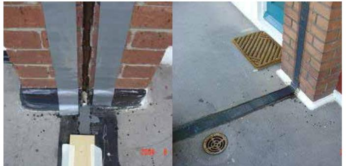
Leaking expansion joint repaired
