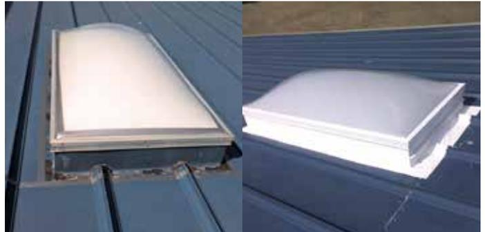
Skylights sealed with waterproofing membrane
