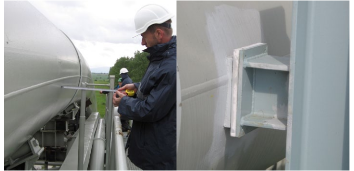
Pipe support bonded
