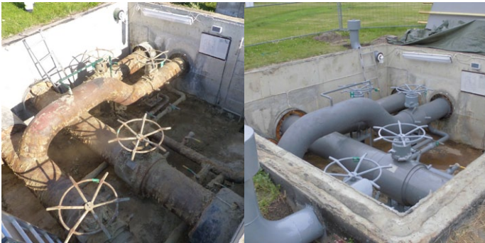
Corroded pipework coated
