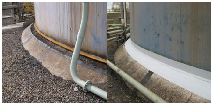
Sealing of tank base
