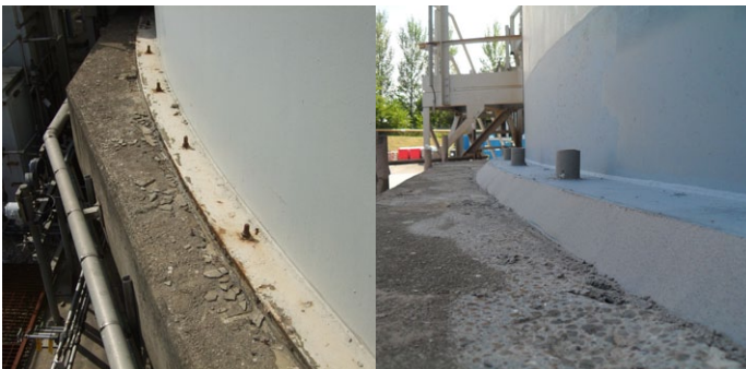
Tank base fillet installed
