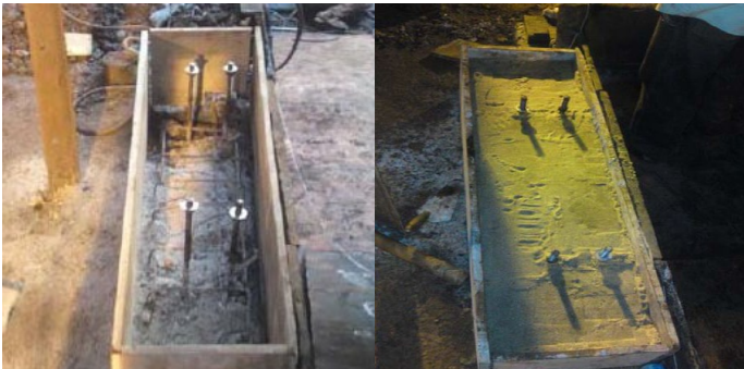
Screen base repaired
