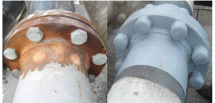
Flange encapsulated for corrosion protection
