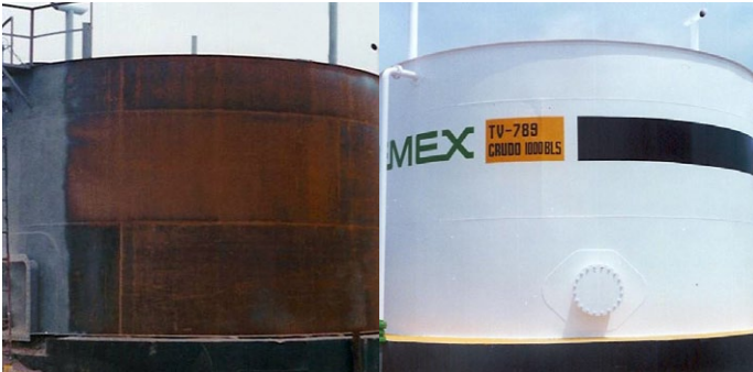
Tank external protected
