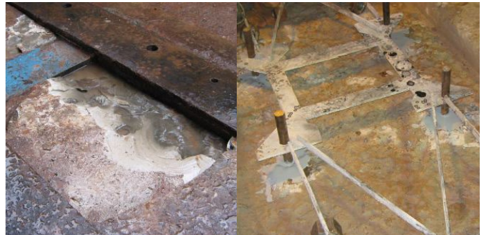
Anchors set on gearbox
