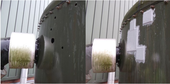
Cold plate bonding on tank
