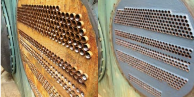
Heat exchanger coated for erosion-corrosion protection
