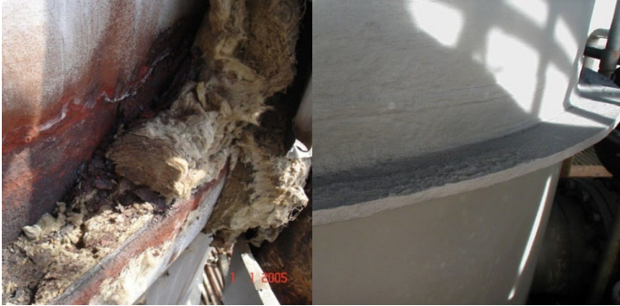
Protection against corrosion under insulation on vessel
