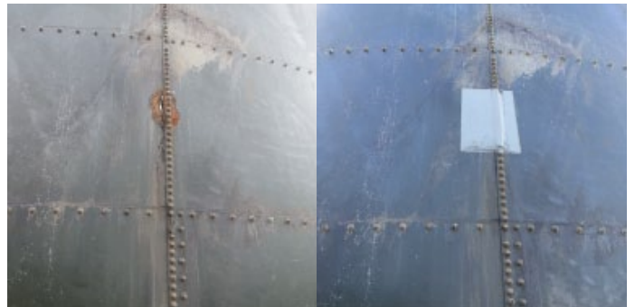
Defect on tank sealed by patching
