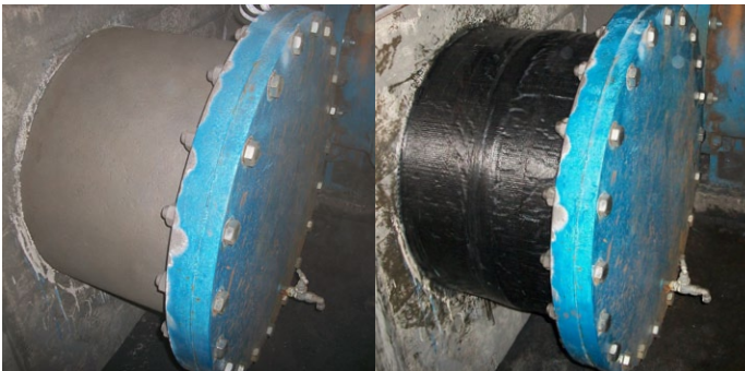
Wrap repair on pipework
