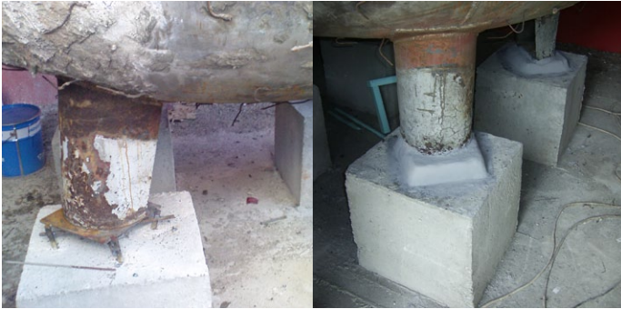
Vessel supports repaired by shimming
