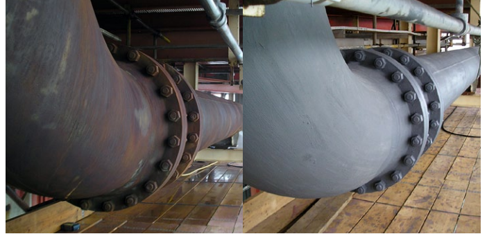
Coating against corrosion under insulation on hot pipework
