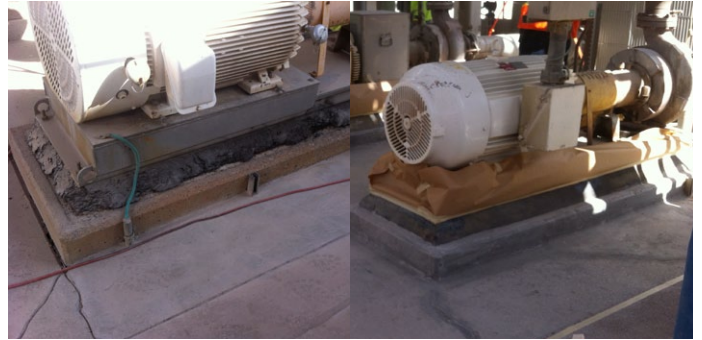
Electrolyte pump base restored
