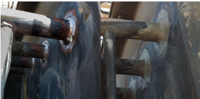
Sealing of leaking pipework
