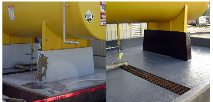
Secondary containment area coated for chemical protection
