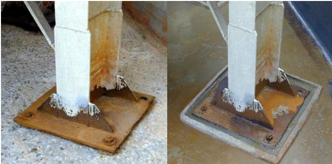
Tank support on chemical containment area secured
