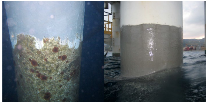
Offshore production platform leg protected
