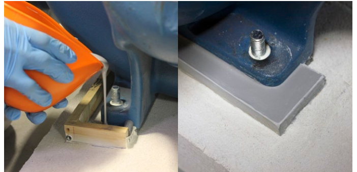
Installation of pump base
