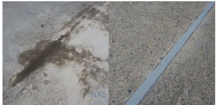
Expansion joint repaired
