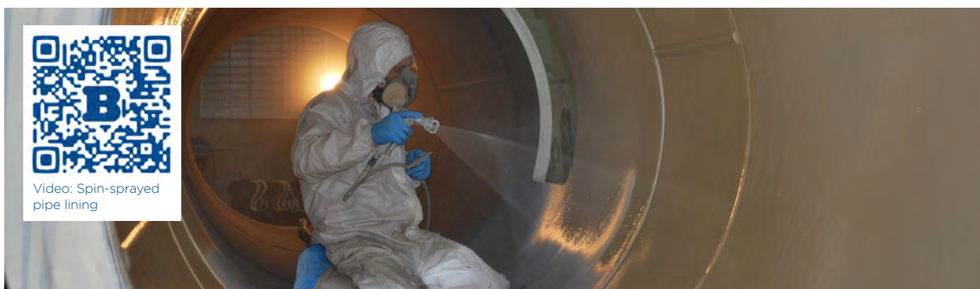
Girth weld covered in a single coat
