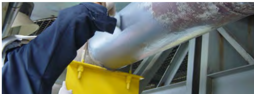
CUI solution applied on-line onto hot contaminated surfaces
