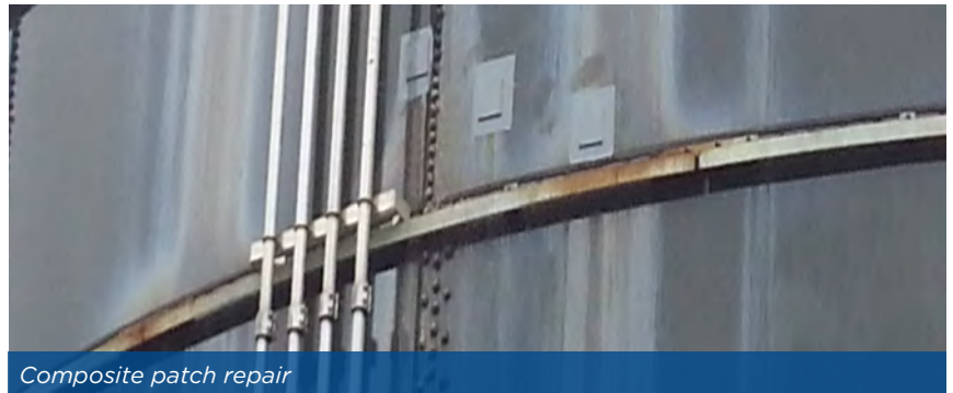
Corroded base
