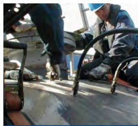
Injection bonding
