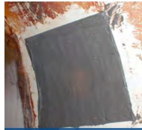
Glass flake lining repair
