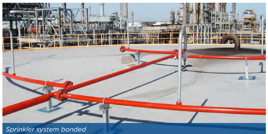
Pipe supports bonded
