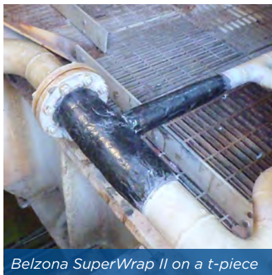
Leaking brinefield pipe
