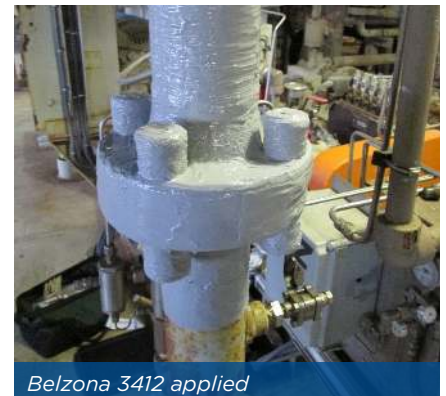
Belzona 3412 applied
