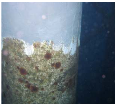
Corroded platform leg
