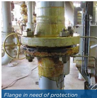
Flange in need of protection
