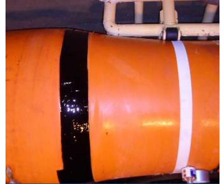
Belzona flexible repair
