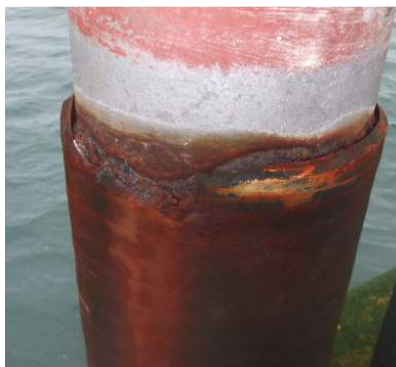
Corroded riser
