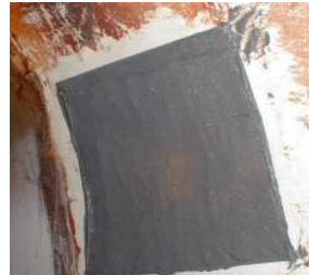
Glass flake lining repair
