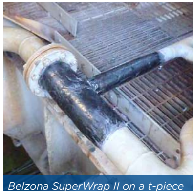
Belzona SuperWrap II on a t-piece
