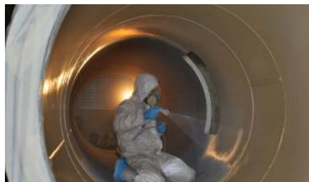
100% solids epoxy protective linings for erosion-corrosion protection
