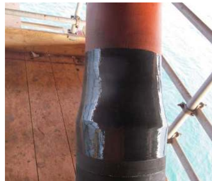
Corrosion repaired and cladding sealed
