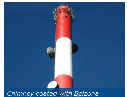
Chimney coated with Belzona
