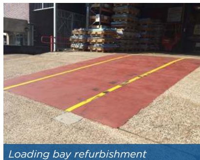
Loading bay refurbishment
