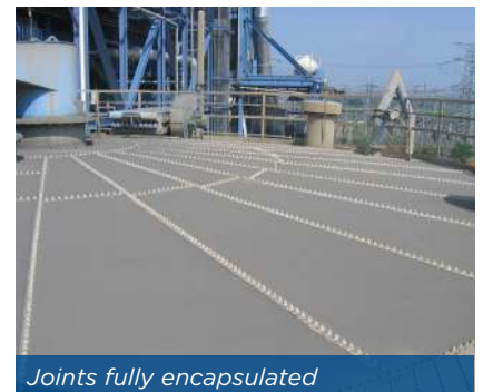
Base sealed with a Belzona coating
