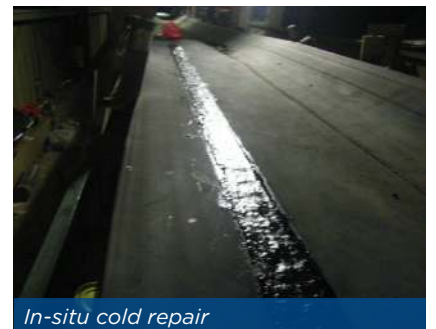
Internal section lined with Belzona
