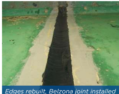
Edges rebuilt, Belzona joint installed
