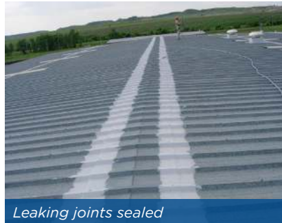
Leaking joints sealed
