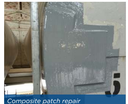
Composite patch repair
