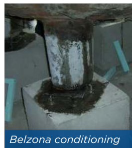
Belzona being applied
