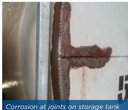
Corrosion at joints on storage tank
