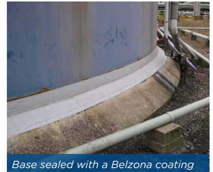
Base sealed with a Belzona coating
