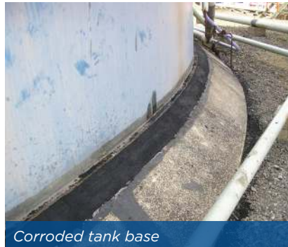
Corroded tank base
