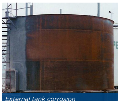
Corrosion at joints on storage tank
