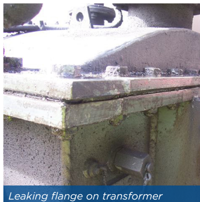
Transformer leaking oil from cracks
