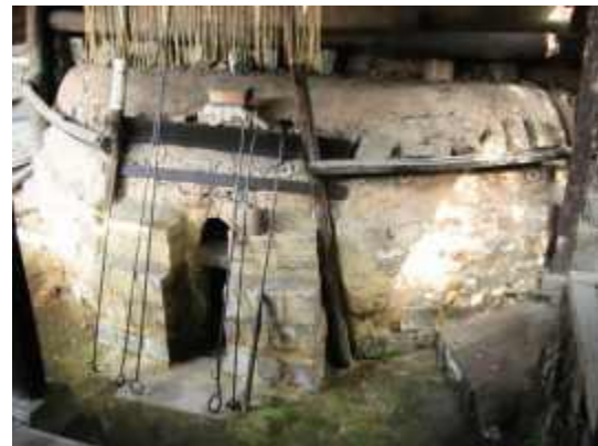
A view of the firebox and the secret chamber with the stirring rods ready to tend the fire.
