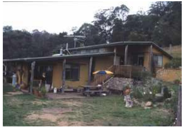
Daniel's hand built house made from adobe bricks was very cool and comfortable in the heat.
