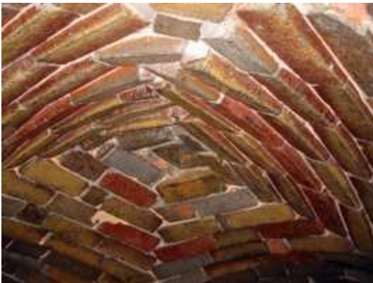
Daniel's amazing brickwork in the domed roof of his woodfired car kiln.
