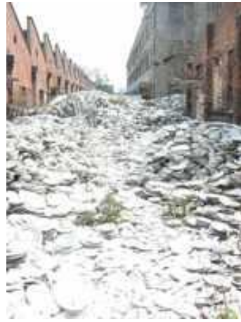
The porcelain pathway between the old and new buildings.
