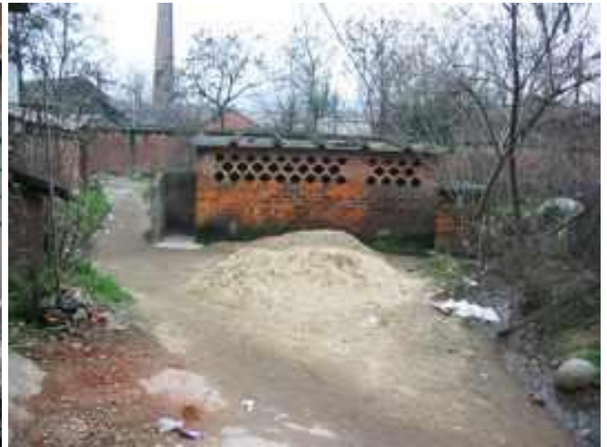
Public latrine for a nearby apartment building. It is emptied daily with buckets into "honey wagons". This is used as "night soil" fertilizer.
