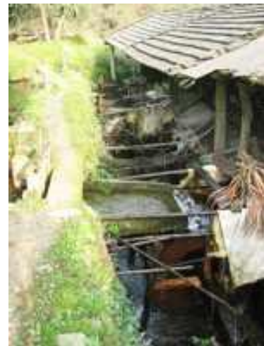
The river water is directed to the water wheels
