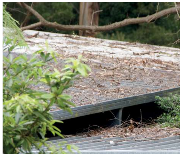
Vegetation located too close to a house poses a threat during bushfire.
