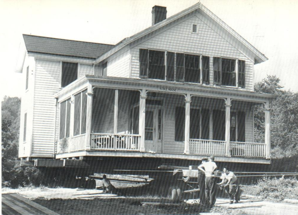
ON THE MOVE. Keble House is moved to the North side of the road.
