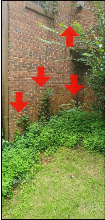
9. potential moisture intrusion
