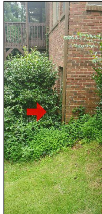
12. potential moisture intrusion
