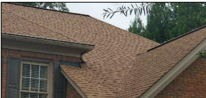
5. Asphalt shingles
