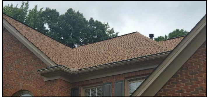
2. Asphalt shingles
