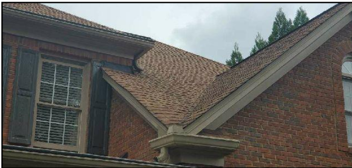
3. Asphalt shingles
