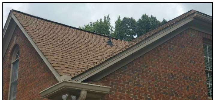
6. Asphalt shingles
