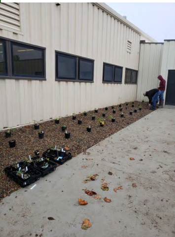
Laying out the plot.
