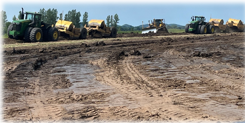
Top Left: Contractor crew building low-profile berms with scrapers and dozer, Pike Co.
