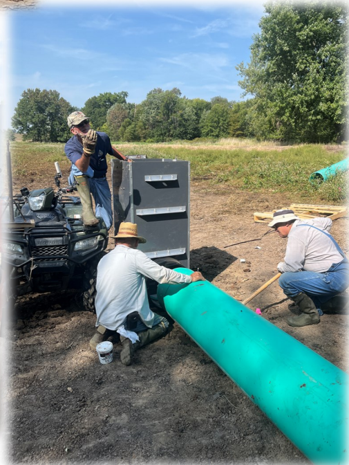
Bottom Right: The one, the only Wetland Emphasis Team 2 setting a water control structure, Adair Co
