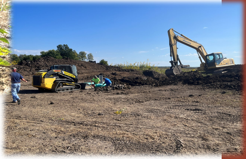
Above and Below: Setting water control structure on new WRE in Lincoln Co
