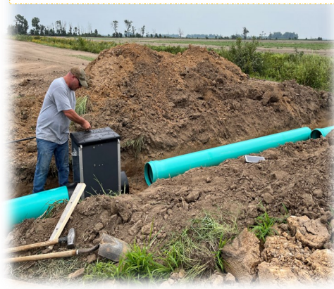
Above/Below: One of the last steps in the construction process is putting in the WCS to help drain or flood WRE pool acres
