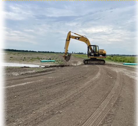
Above/Below: One of the last steps in the construction process is putting in the WCS to help drain or flood WRE pool acres
