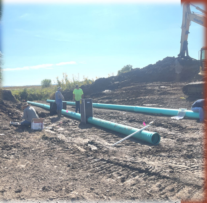
Above and Below: Setting water control structure on new WRE in Lincoln Co
