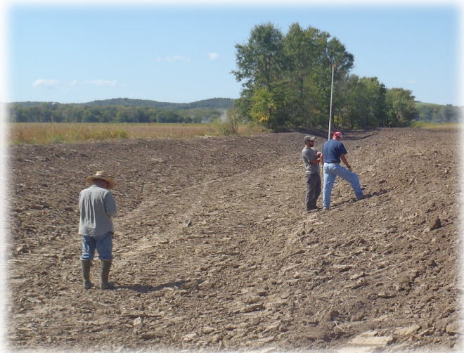
WET2 conducting checkout on Lincoln Co easement
