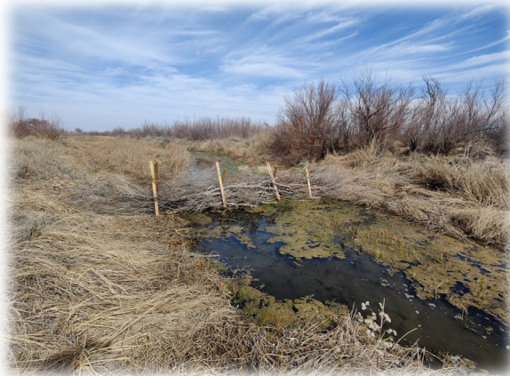
Post-construction monitoring of a beaver dam analog (BDA) on a ranch in south-central Kansas from my time as a Wildlife Biologist
