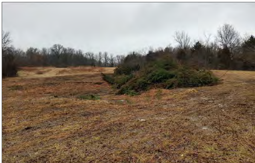
A section of brush cleared by chainsaw, skid-steer, and elbow grease.
