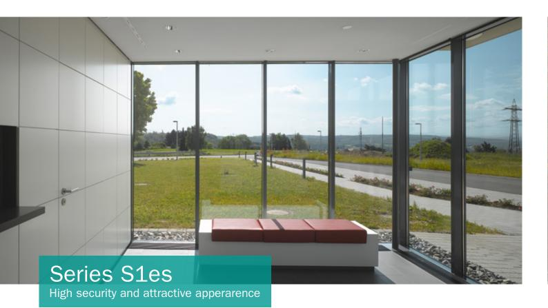
The S1es series aluminum facade offers combinable protection against forced entry, bullet and blast up to the highest resistance classes. The high-security components are integrated invisible inside the profiles. The S1es series can be seamlessly combined with the Schüco FWS façade system.
