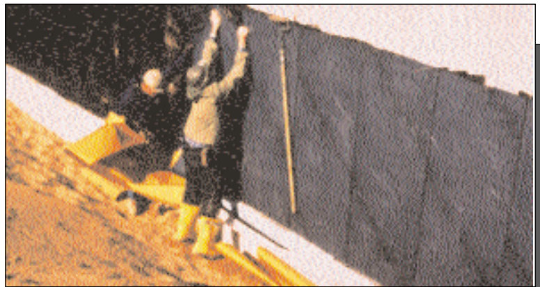
Below-grade Concrete Wall Installation
