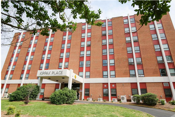
Kippax Place after renovation. Photo courtesy of Community Housing Partners
