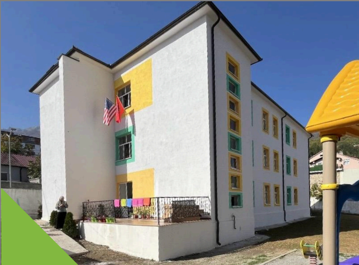
Kindergarten No 1 Reconstruction, Bajram Curri 2024
