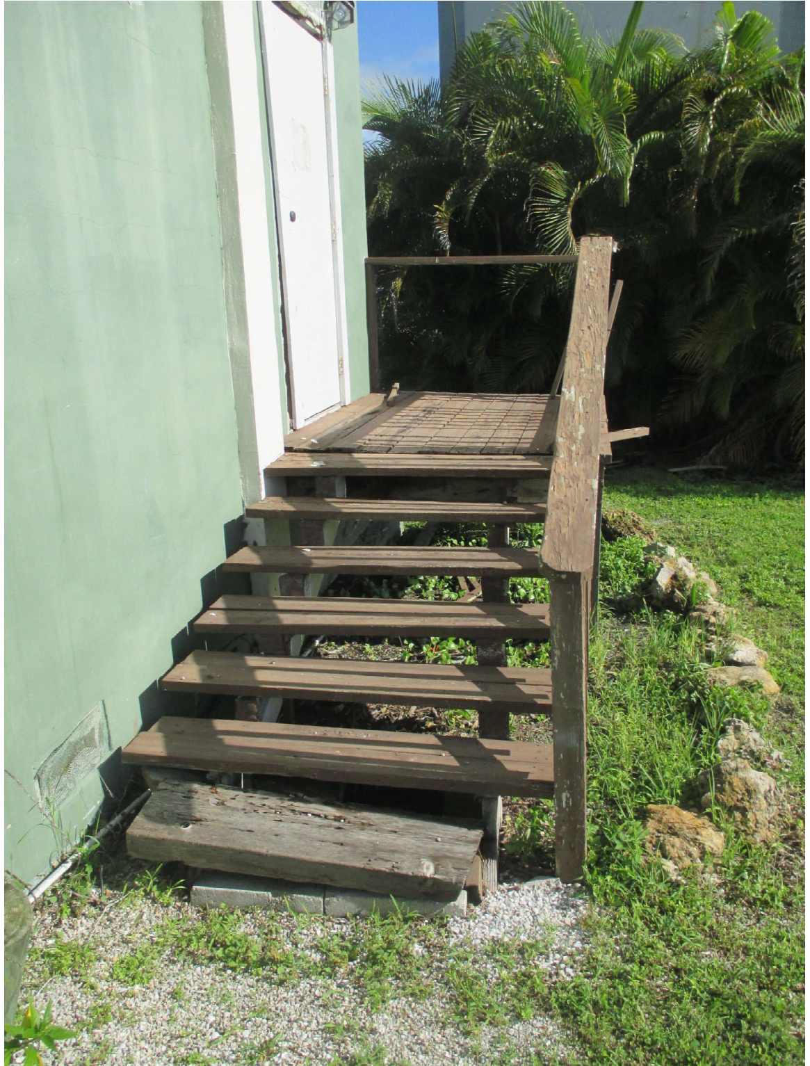
Photograph 14 East Facade Deteriorated Wood Stair Requiring Replacement on New Footings
