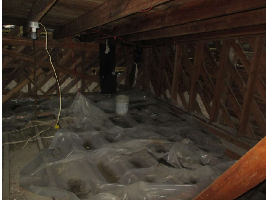
Photograph 5 Plastic Membrane in Attic Over Ceiling
