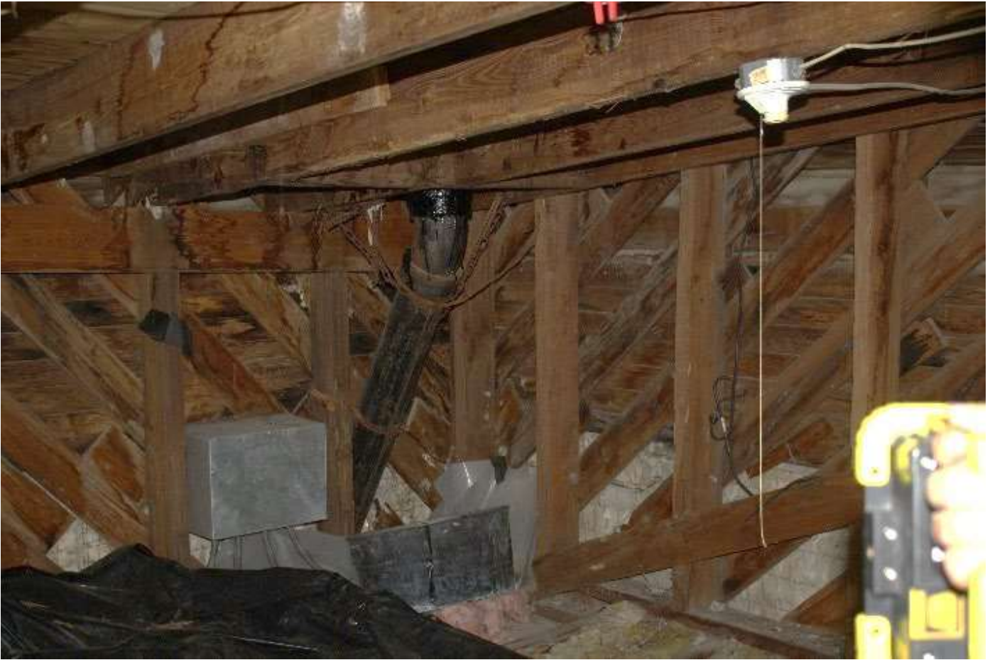
Attic area showing roof drain and plastic
