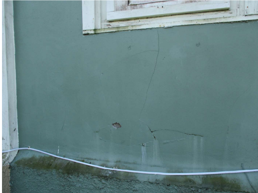
Photograph 19 Northwest Corner Cladding Spall
