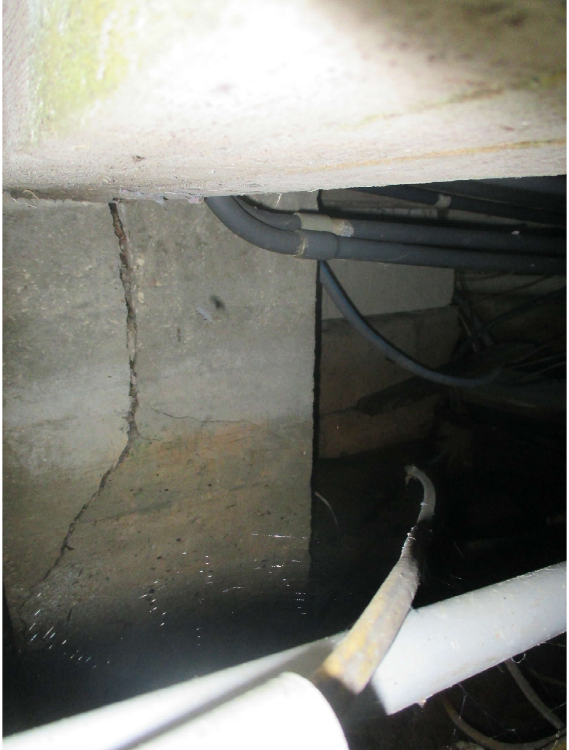
Photograph 13 Northeast Foundation Pier Cracked
