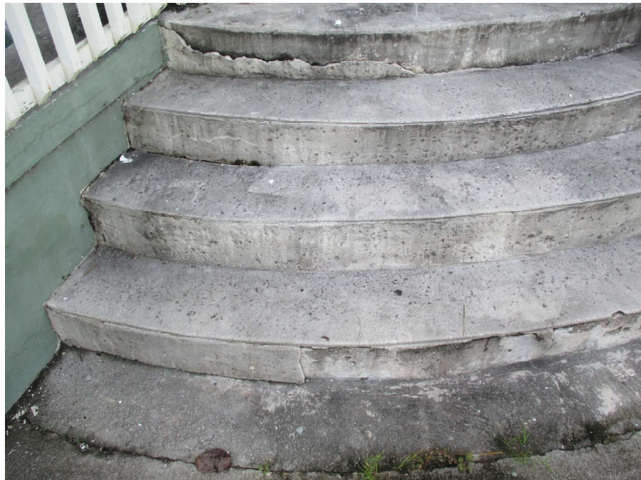
Photograph 16 West Façade Entry Steps - Topping Deterioration
