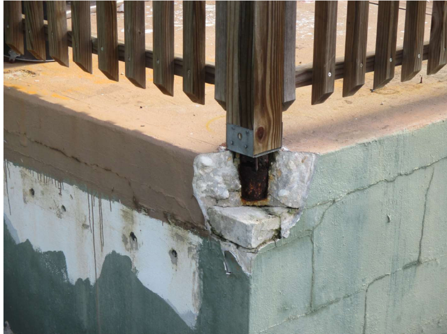
Photograph 17 South Façade Entry Handrail - Base Deterioration
