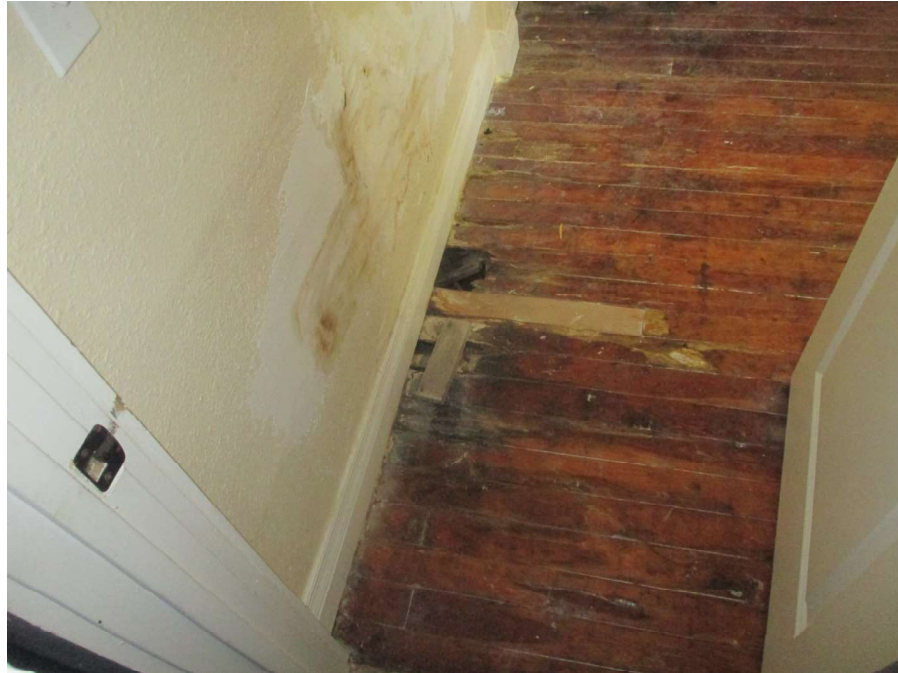
Photograph 7 Water Damage Due to Plumbing Leak
