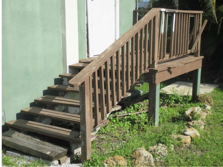
Photograph 15 Failed Handrail and Bearing On Grade
