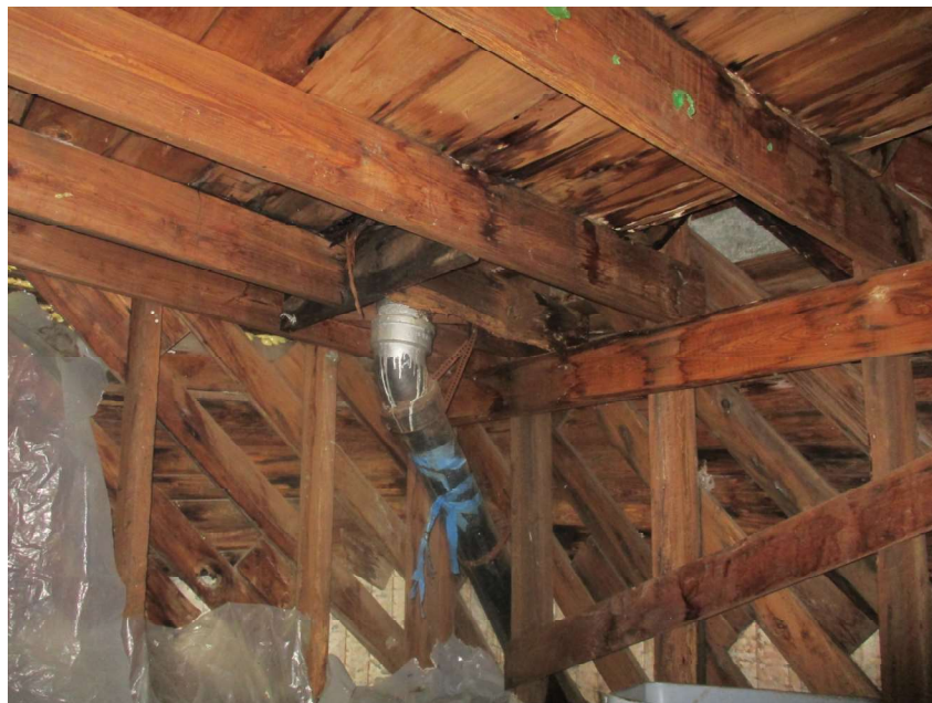
Photograph 4 Deteriorated Roof Framing at Drain
