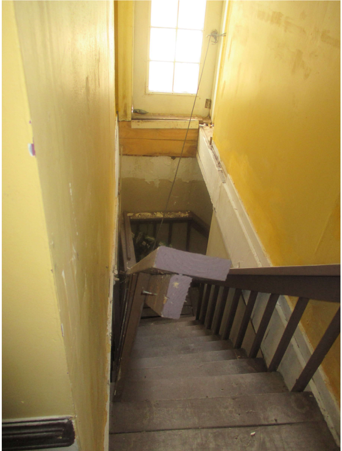
Photograph 11 Failed Stairs and Handrail at Northeast Corner
