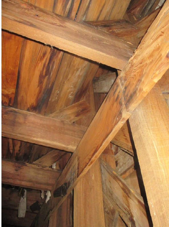
Photograph 3 Parapet Knee Brace
