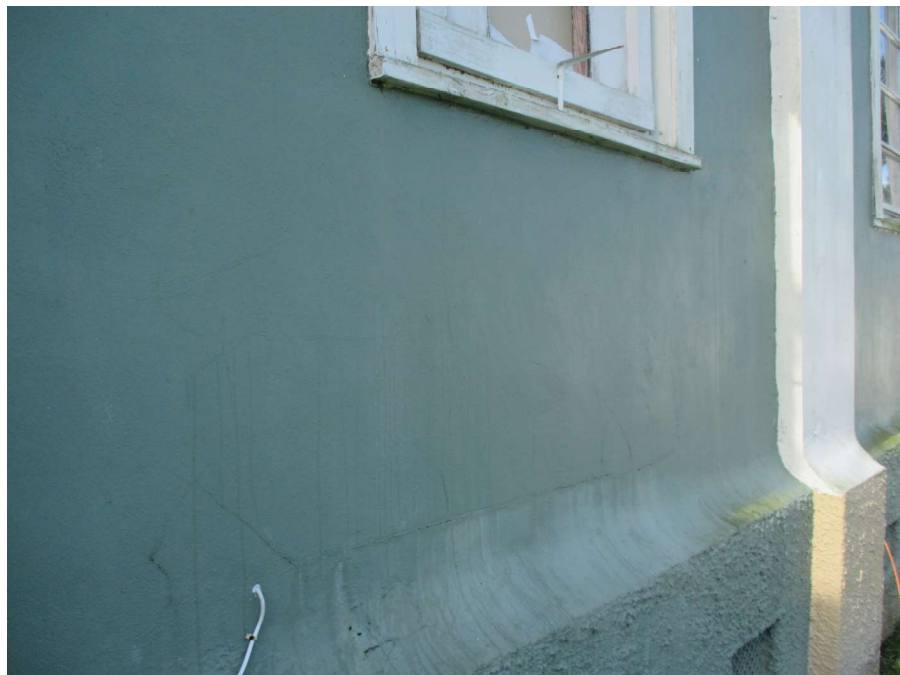
Photograph 20 Cladding Crack at First Floor Joint
