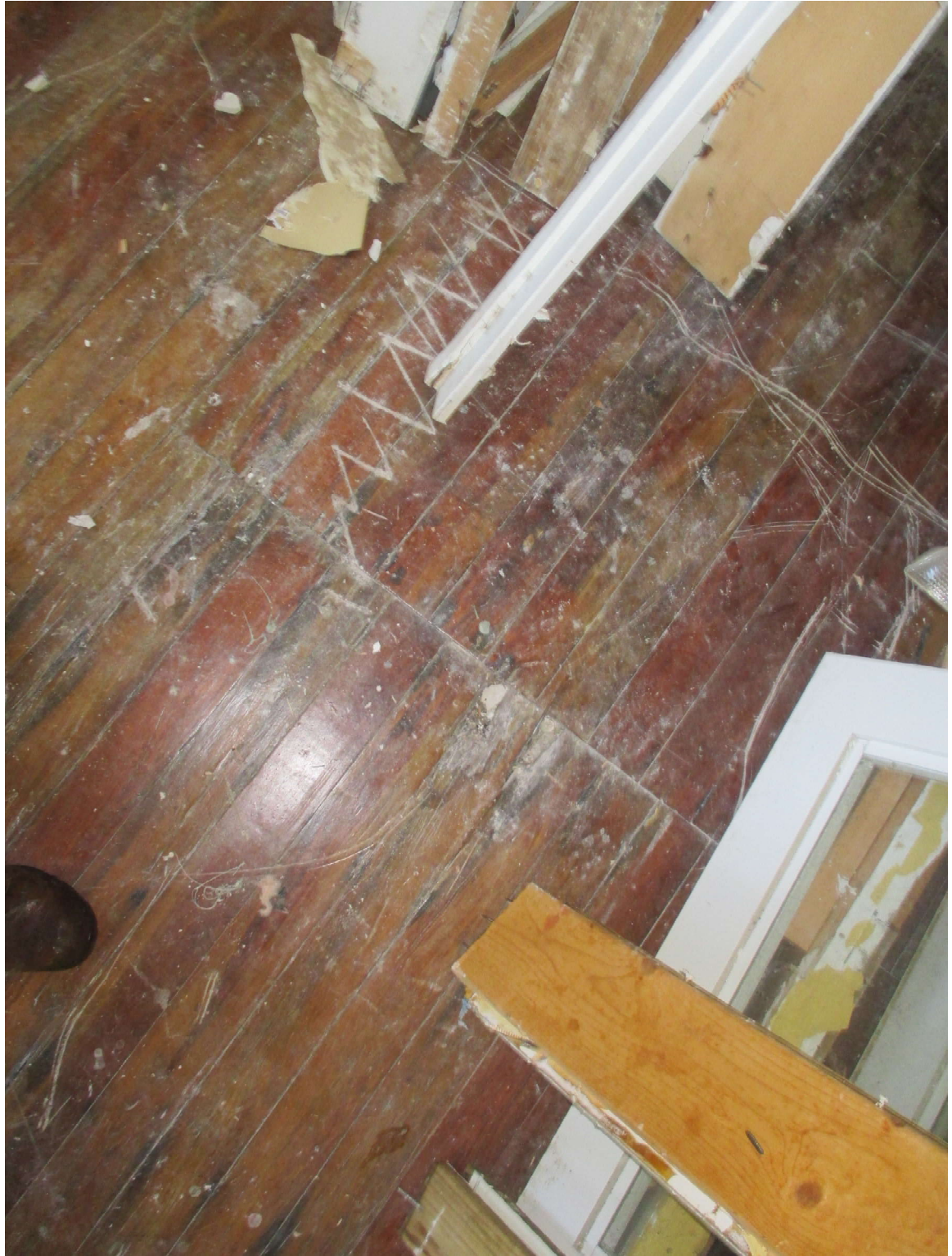
Photograph 12 Deteriorated First-Floor Decking
