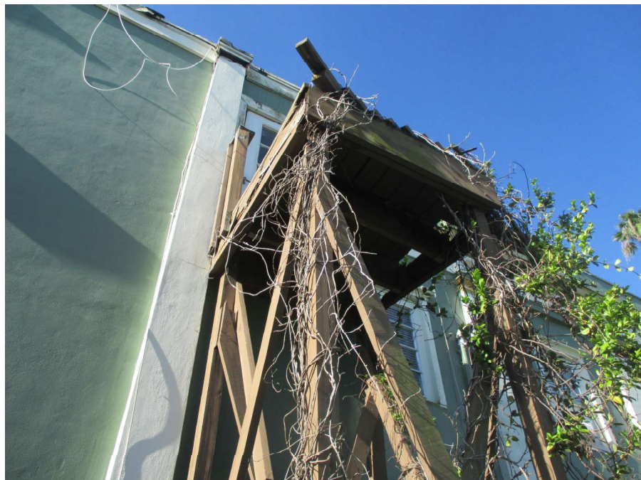
Photograph 18 North Façade Entry Deterioration
