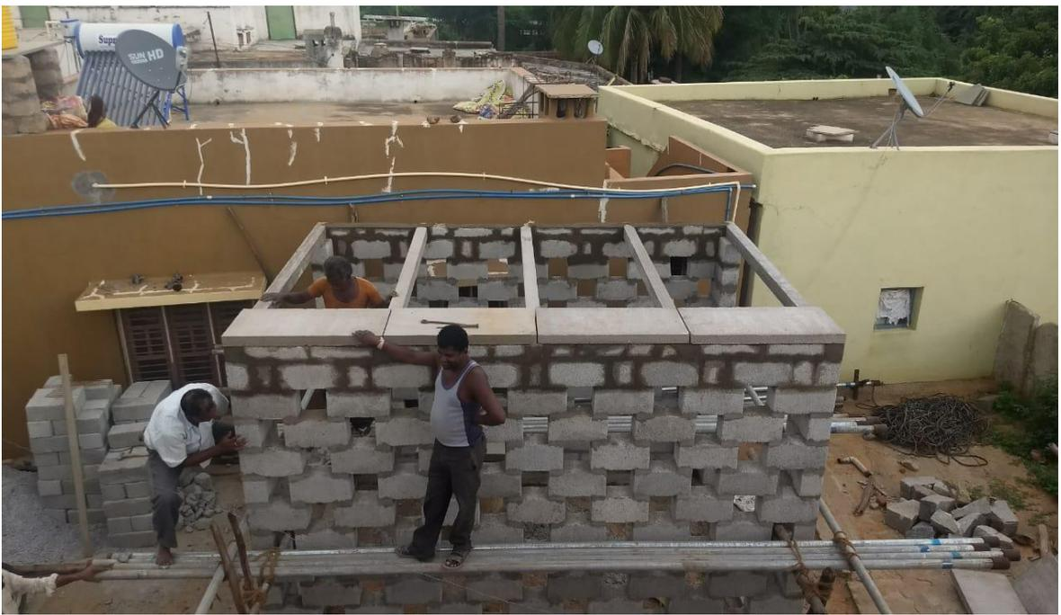
**Prototype of RCC panel and rafter roof technology at Namagondlu**
