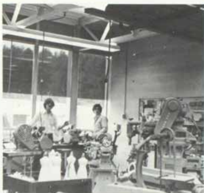
Machine shop looks more like a hazard area than a classroom.
