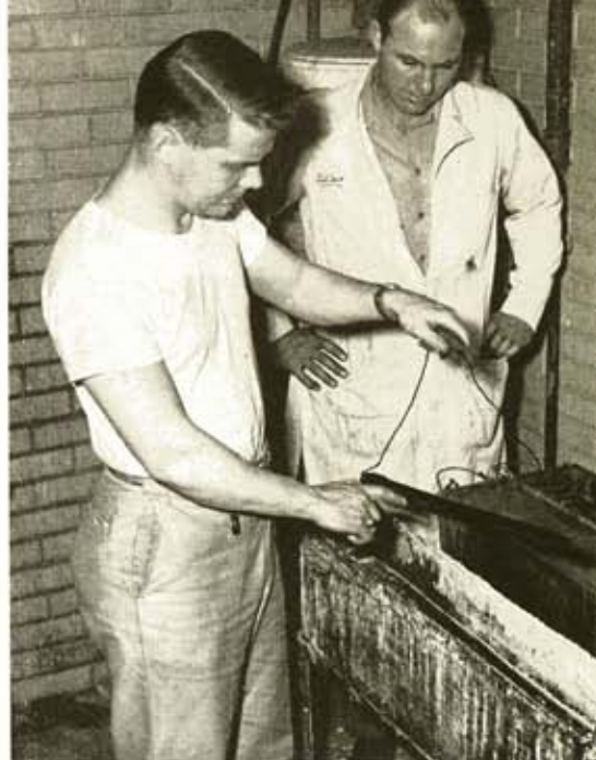
Instructor and student inspect a re-blued barrel before final oil bath.
