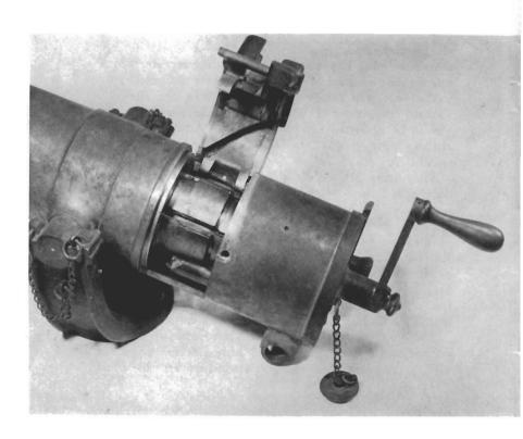
bered for the 45/70 U.S. Service cartridge and the Martini cartridge of 45 caliber for England. A further change was the doughnut shaped Accles drum feed. It held 104 shots and was linked to the main rotating shaft of the gun through a system of cogwheels.
