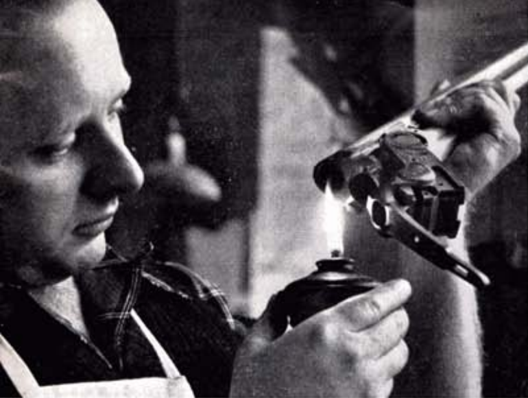
Smoking breech face of barrels shows bearing points.
