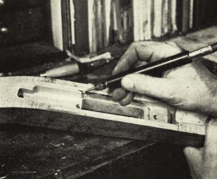
Cutting away tiny shoulders and high spots in final inletting, Kishel uses Do-All grinder with high speed burr.
