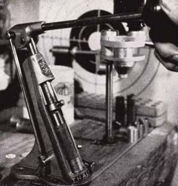
Primers are seated in de-capped shell by plug which pushes case on new cap.
