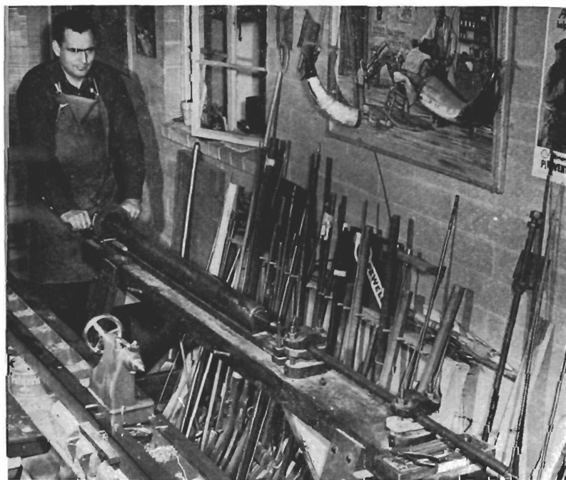
In his Albuquerque shop, riflesmith Dick Hicks cuts rifling grooves in barrel blank moving cutter by hand.
