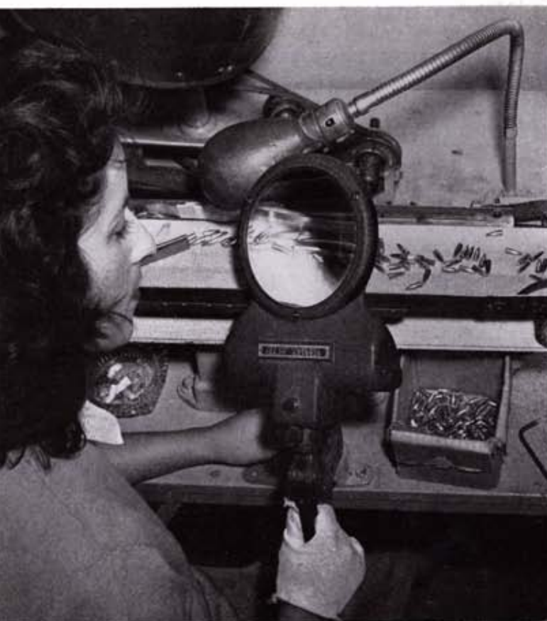
Final inspection with magnifying glass is made of each bullet on moving belt just before packaging for shipment.
