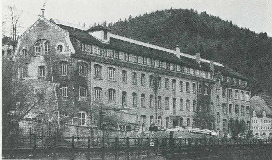
This much is left today of the Schweden-bau, where all Mauser handguns were made from about the turn of the century on. The fitting room was at attic level, with production departments on the first 3 floors.
