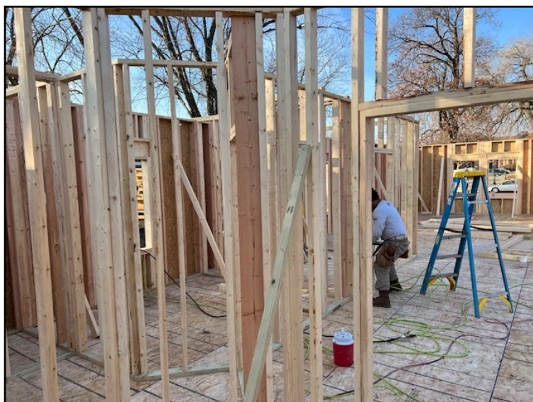
Photos taken of the construction progress on December 21 (Brandon Wilsey)
